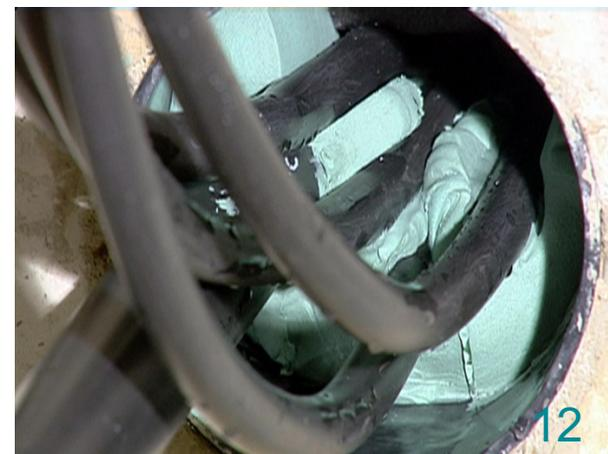
Lift the cables and apply the 2100 Aquastop with a suitable injection tool around the cables.
