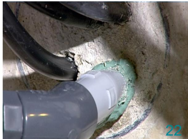
A cable can be removed from the duct with the same procedure. Remove the cable → Apply 2100 Aquastop and Mortar WR or FR.
