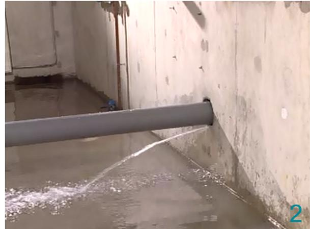
2 The sealing system can be applied while the duct is leaking.
