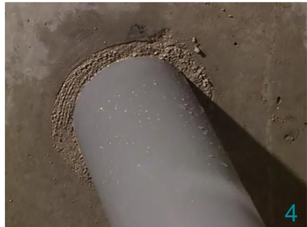
Mortar FR for ducts with Flame retardant properties
