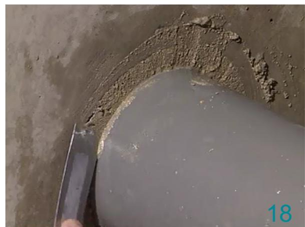
Smoothen the surface of the mortar by using a putty knife and a small amount of water.
