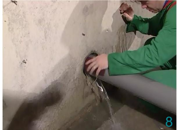
Adhesion can be improved when pipe and duct are pre-applied with 2100 Aquastop.
