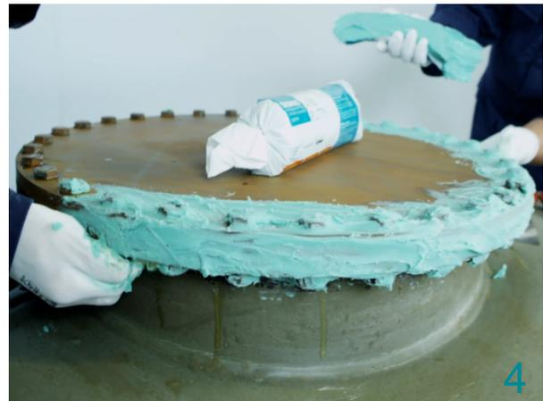
Apply a thin layer of 4100 Putty on the entire area around the bolts.
