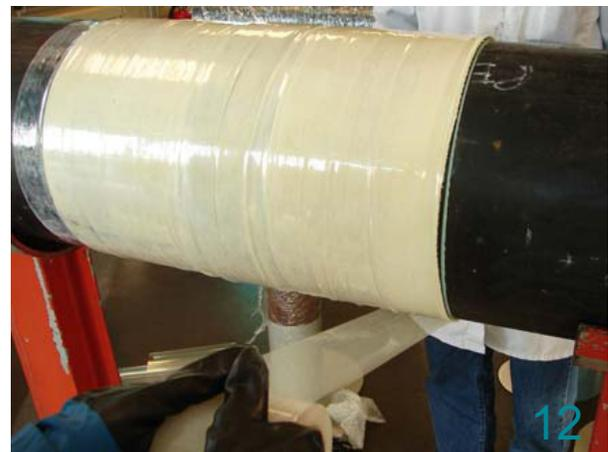
Outerglass Shield should overlap the factory applied coating approx. 100mm.
