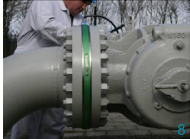
The rectangular cut in the ratchet strap enables tightening the clamp.
